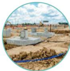
Interconnection pipe rack foundations
