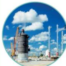
First equipment being set (acetylene reactors in Cracker area)
